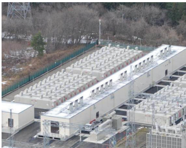
Image: Minami-Soma Substation in Japan Source: www.toshiba.co.jp/about/press/2015_04/pr2101.htm
