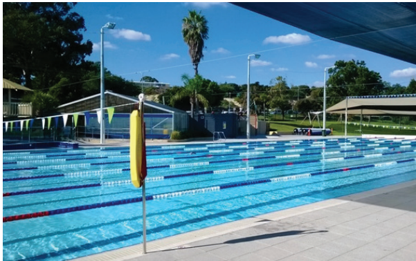
Image: Fremantle Leisure Centre's 50m pool heated with shallow aquifer geothermal and cogeneration (Source: City of Fremantle)
