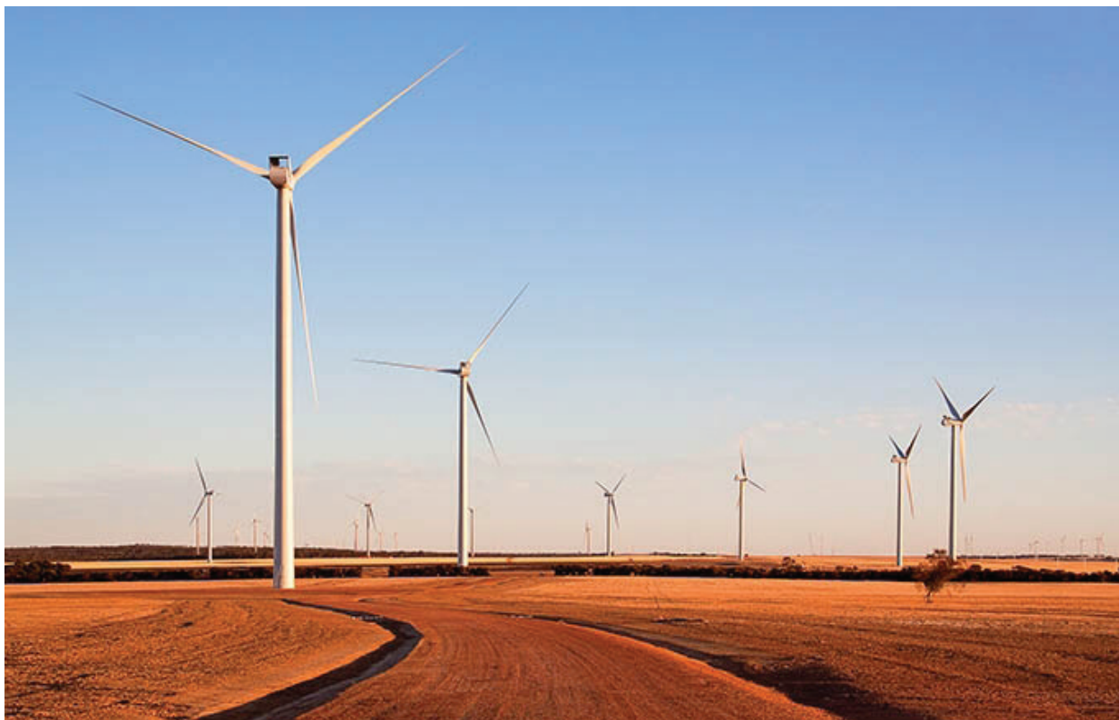
Image: WA's 200MW $750m Collgar Wind Farm, operating at a stunning 50% capacity factor (Source: Collgar Wind Farm http://www.collgarwindfarm.com.au/about-us/ )
