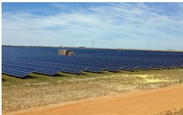
Australia's first utility scale solar farm opened in Greenough, WA in 2012.
