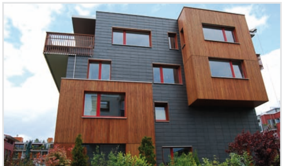
An example of innovative high density design and materials used in the Vauban Quarter of Freiburg, Germany
