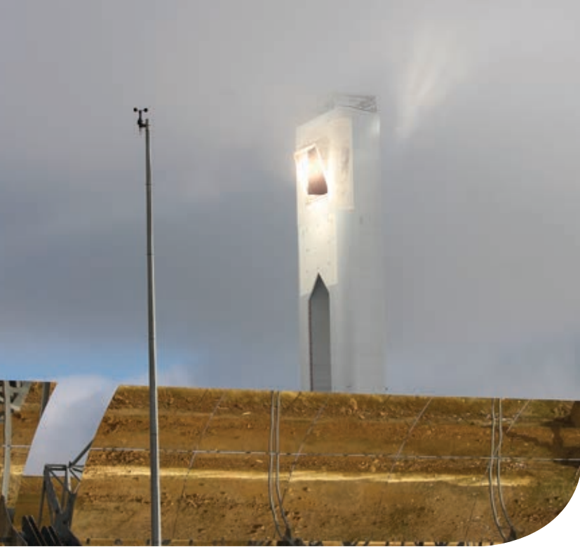
Abengoa's Planta Solar 20 plant, Sanluca la Mayor, Spain (Image: Scott Ludlam)
