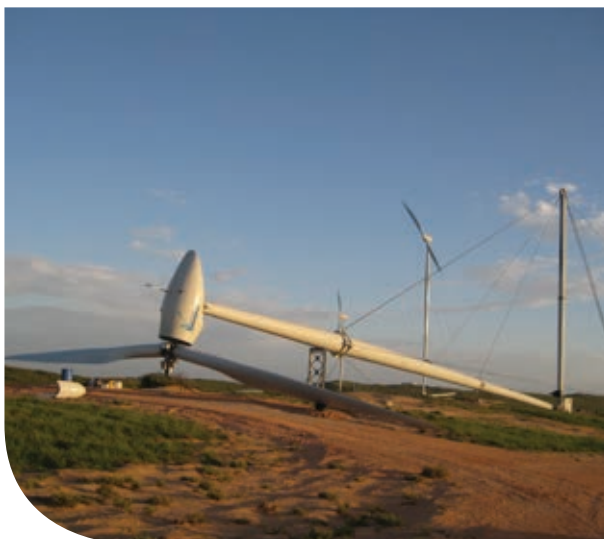
Turbine being lowered for maintenance at Coral Bay wind farm Photo Credit: Brendan Ryan at http://ramblingsdc.net/Australia/WindWA.html#Wind_power_generation_in_WA
