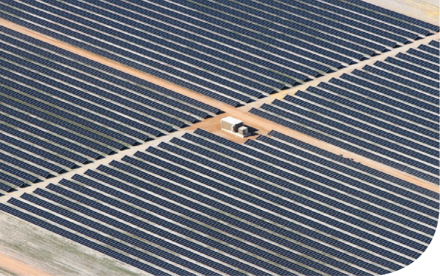
Images top and right: Greenough River Solar Farm
