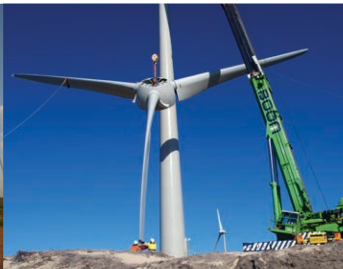
Denmark community wind farm under construction (2012) Photo credit: www.skyfarming.com.au/normal.dcw.htm#turbineinstall/turbineinstall_4.htm
