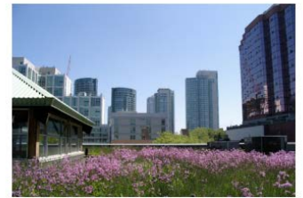
Image: Green roof on Toronto's Mountain Equipment Co-op store.
