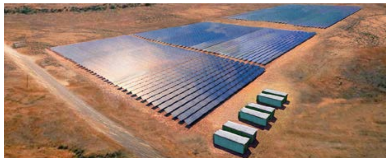
Image: An Artist impression of the 100-megawatt solar and 100-megawatt storage facility to be built in South Australia (Source: AFR 8 September 2016)
