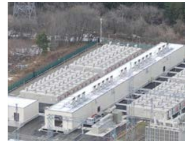
Image: Minami-Soma Substation in Japan Source: www.toshiba.co.jp/about/press/2015_04/pr2101.htm
