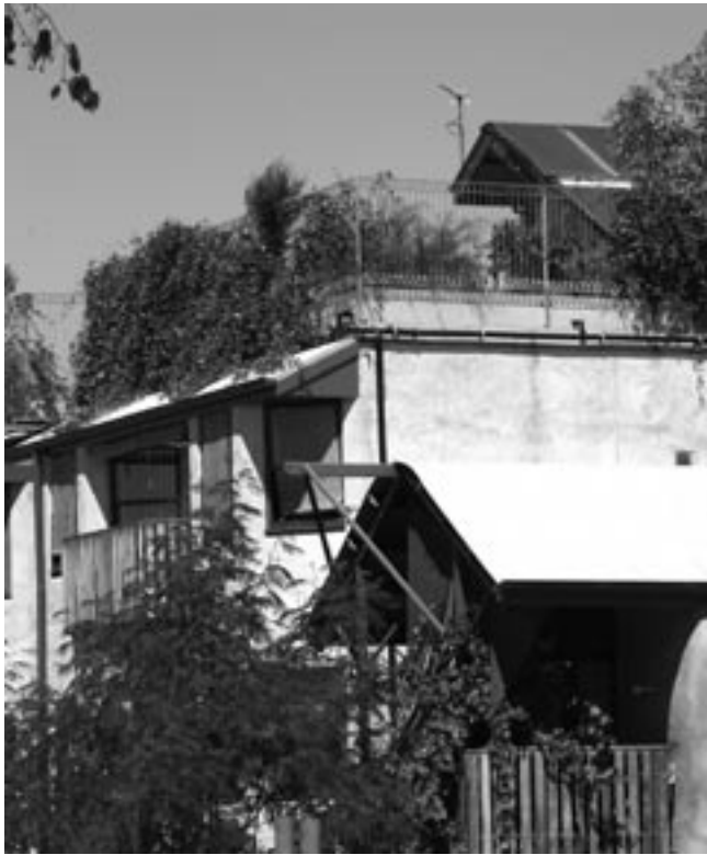
Rooftop garden and solar collectors at Christie Walk Eco-village, Adelaide. www.urbanecology.org.au/christiewalk
